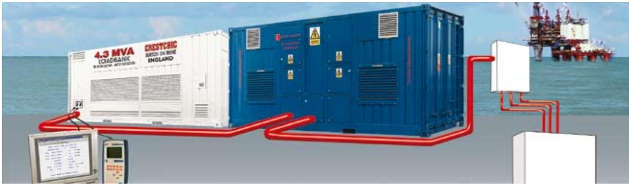
Typical test used for proving power on an oil production platform
